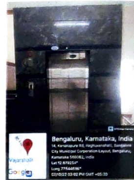
Lift-2 at New Block Exit
