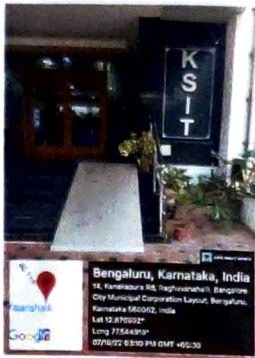
Ramp at New Block Entrance
