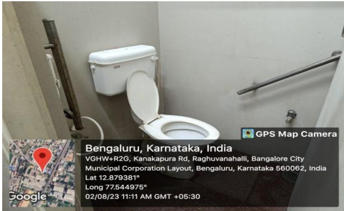
Washroom facility for differently abled
